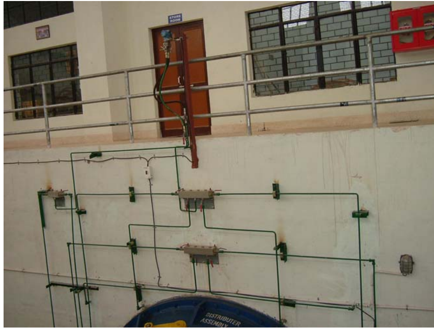
Figure 8.4 – Upward sloping pipes and valves for purging
