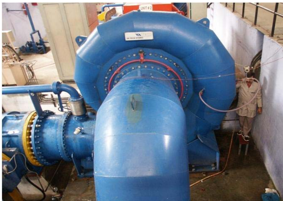
Figure 8.2 – Illustration of pressure taps in vertical steel spiral case
