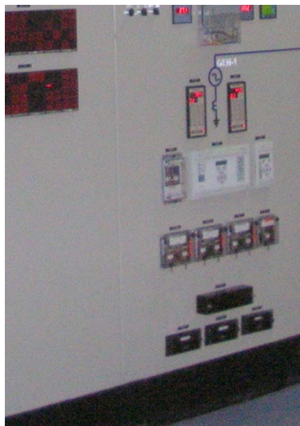
Figure 9.2 – TTB (shown with cover in place) fitted on the front of a control panel
