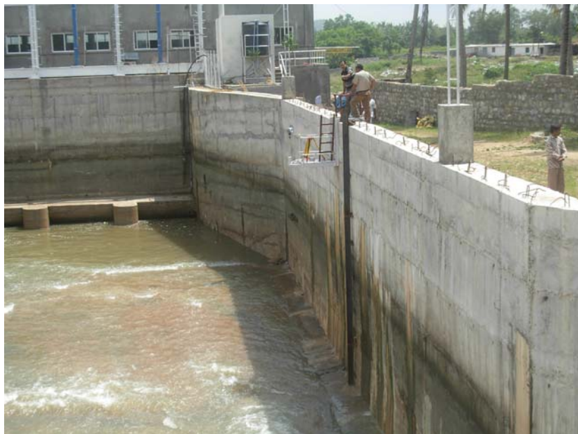
Figure 7.7 – Guide-rail fixed to the channel wall for guiding movement of ADCP trolley
