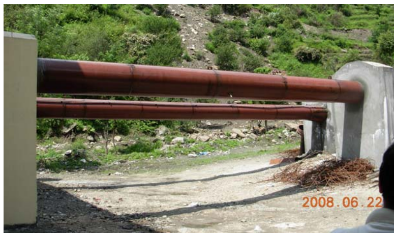
Figure 7.4 – Adequate lengths of penstocks left un-embedded
