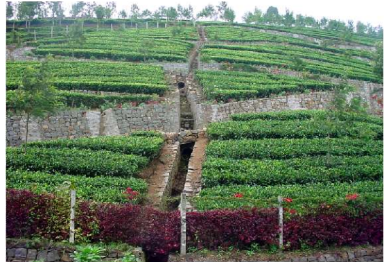
Vertical drain in tea plantation for safe disposal of runoff in the Nilgiri hills
