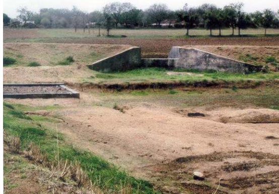
Recharge filter— A cost-effective technology for augmenting groundwater in arable and non-arable lands in arid and semi-arid regions of Gujarat and Rajasthan
