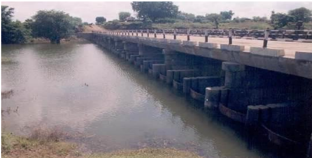
Fig.2 – Bandhara /Barrage Structure constructed on Addan River, Distt. Yawatmal, Maharashtra (MoRTH, 2017)
