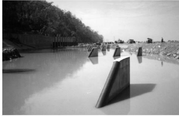
Fig.1 Tapered submerged vane being used in river Kosi in Nepal (Sharma, 2016).
