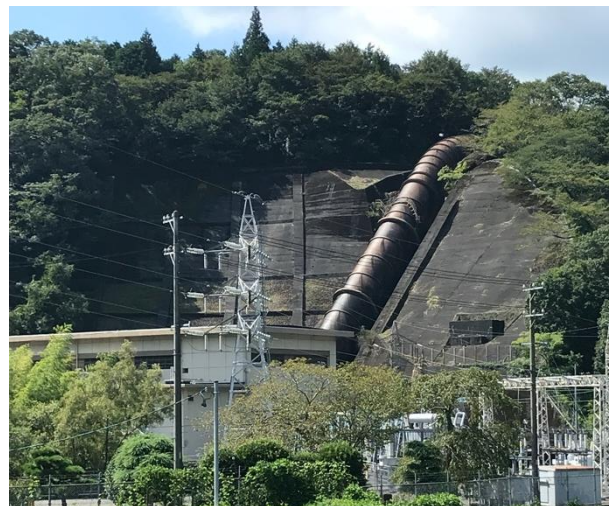
Figure 6 Kawaguchi Power Plant
