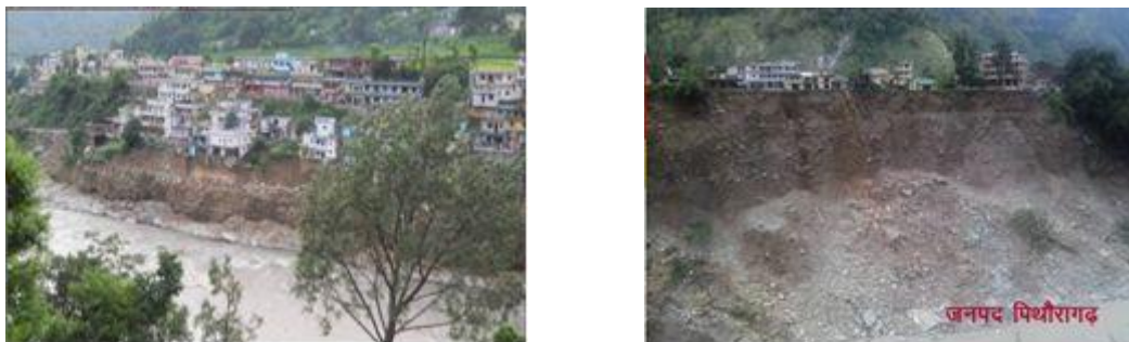
Fig. 4: Damages in District Rudraprayag and Pithoragarh during 2013 flood
