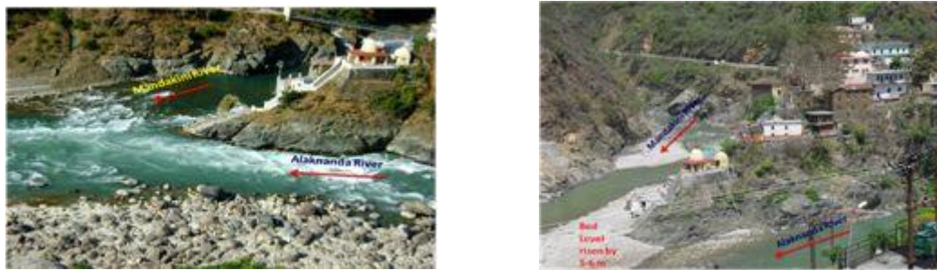
Fig. 3: Confluence of river Mandakini and Alaknanda at Rudraprayag, before and after June 16, 2013
