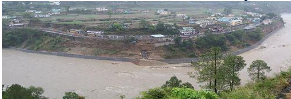
Performance of Defense Structures at Rudraprayag District
