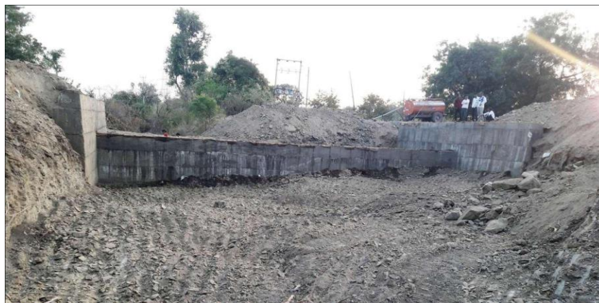
Figure 2: Cement Nalla Bunds
