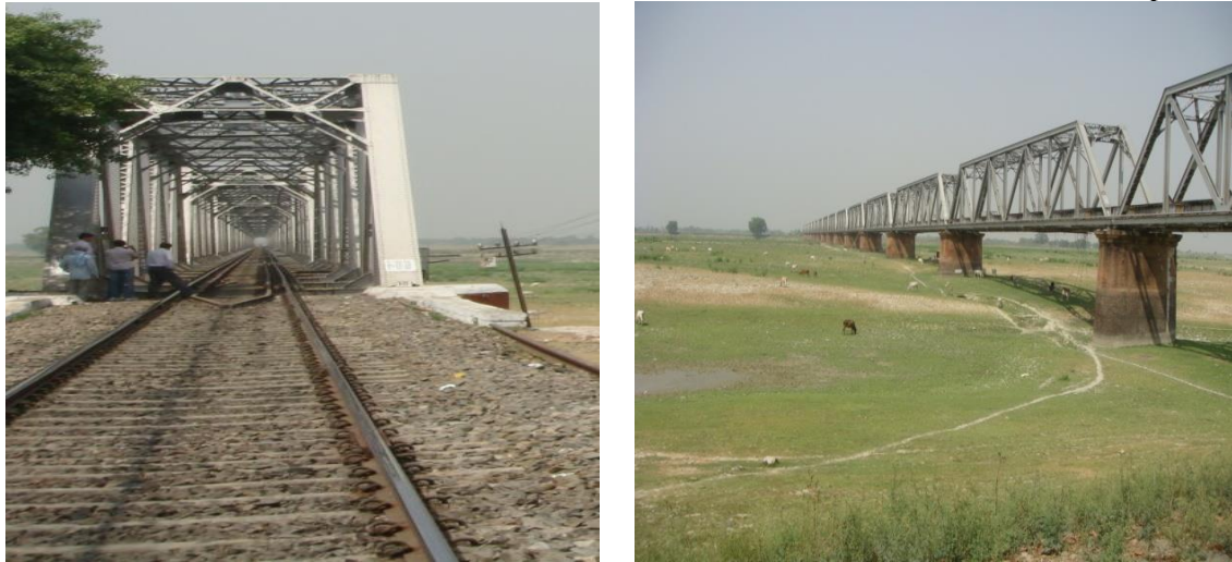
Figure 1: Photographs of Existing Kosi rail bridge near Kursela in Bihar, India
