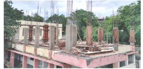
Construction in Progress
