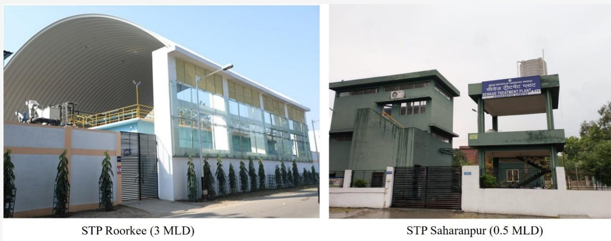
Figure 14: IITR Sewage treatment plant
