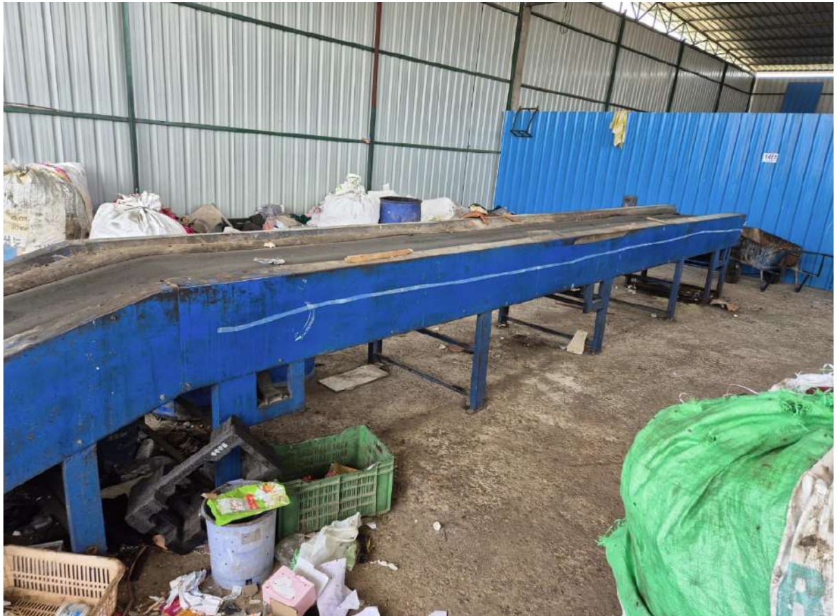
Figure 1 A photo from the SWM facility site
