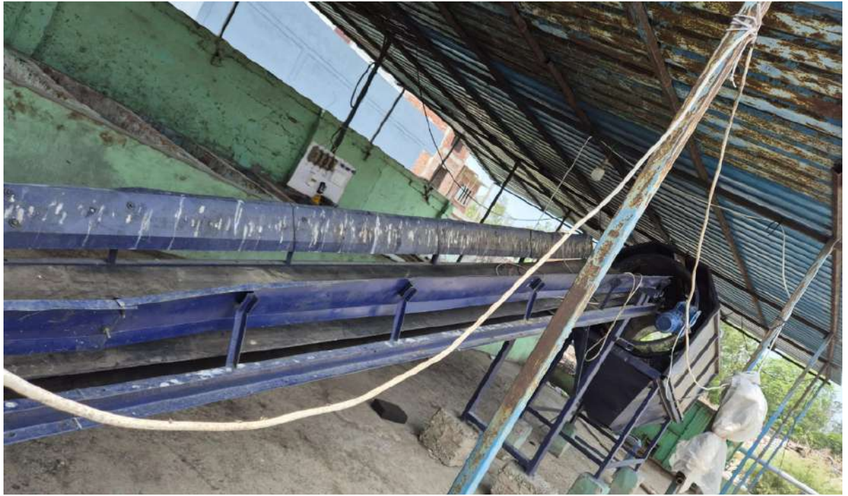
Figure 2 A photo from the SWM facility site
