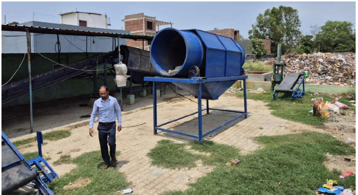
Figure 3 A photo from the SWM facility site
