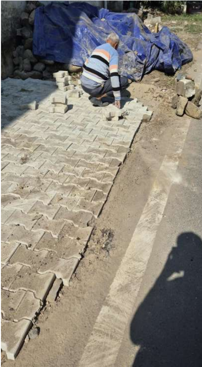
Figure 10 Photo showing continued paving in some parts of the campus
