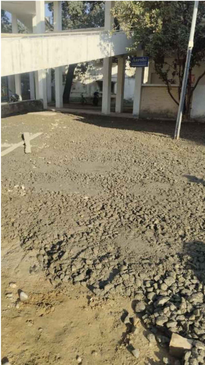
Figure 8 Photo showing continued paving with base concretization in some parts of the campus
