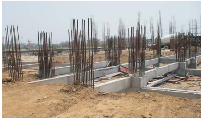
Academic Complex Construction in progress
